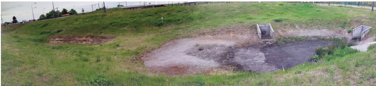
PHOTO 12.6 Swale with overflow option along road in the Netherlands
