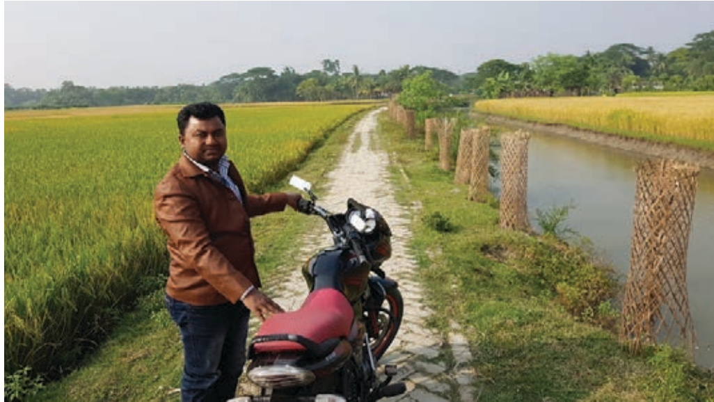
Road created with excavation material from drainage canal in coastal Bangladesh
