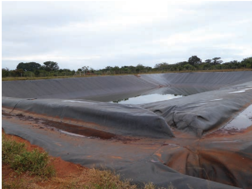
PHOTO 8.4 Borrow pit lined with geotextile, Mozambique
