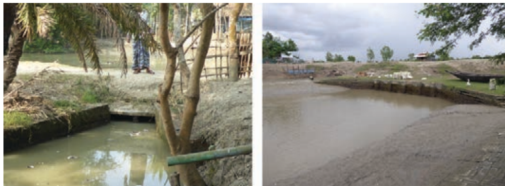
PHOTO 5.8 Use of turfing combined with jute netting
